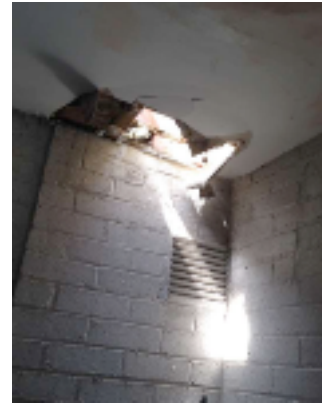
The Willows: Examples of defects Top: ceiling damaged by roofer Visible gap in chimney flashing Vent pipe replaced where penetrating roof but existing hole not repaired Centre: poor workmanship: sundry leaks, incomplete lining to roof Bottom: leaking replacement downpipes, possibly undersized, and displaced leak guard Unfixed and poorly installed soffit
